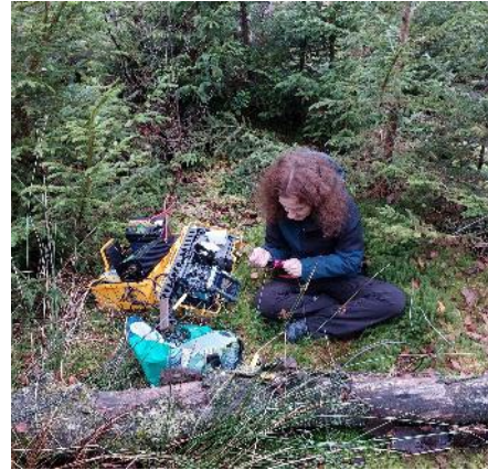
Splicing the fiber optic cable at W6 (2022-11-05)
