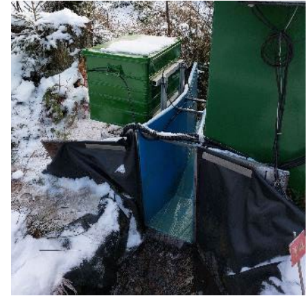
Ultima XT DTS setup next to W14 (2022-12-11)
