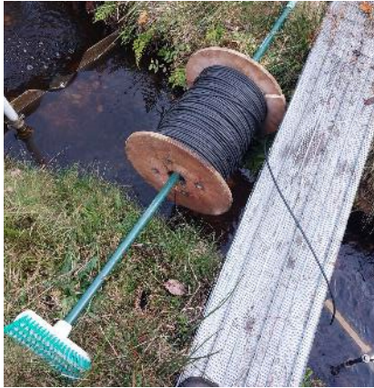
Installation of fiber optic cable at W14 (2022-10-29)
